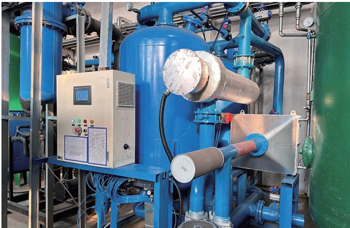
Zero Air Loss Blower Type Suction Dryer
